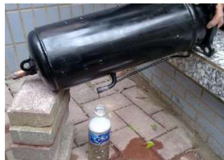
Figure 6-2.5: Draining oil from a compressor
